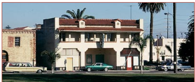
Knights of Columbus building in 1973 when Figueroa Street was still open to vehicles.
